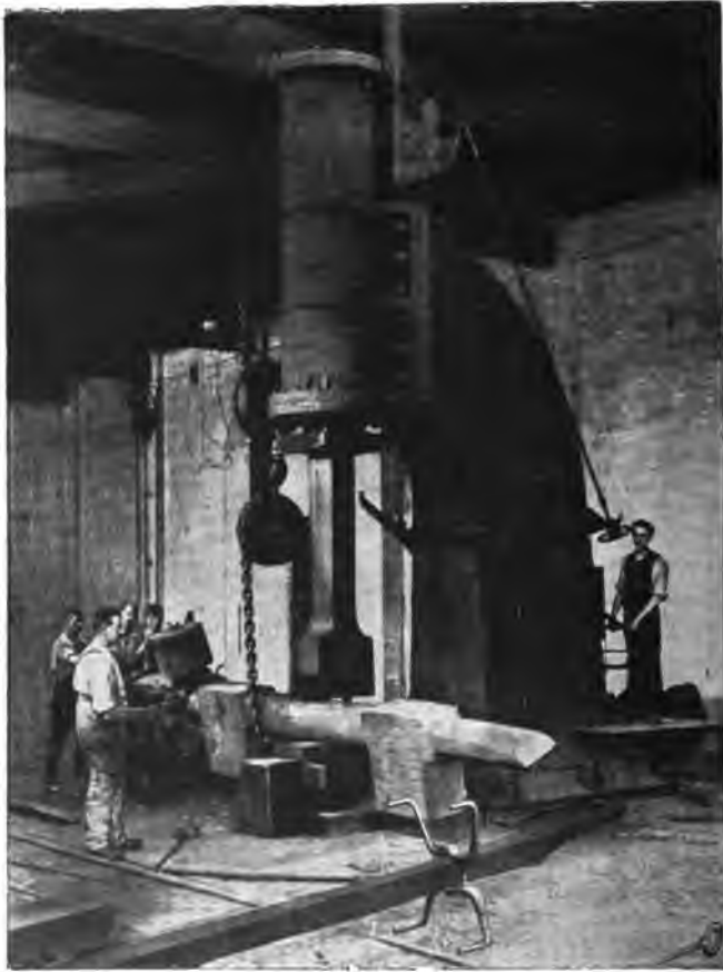
FIG. 414.—Making Double-throw Crankshaft Forging.
